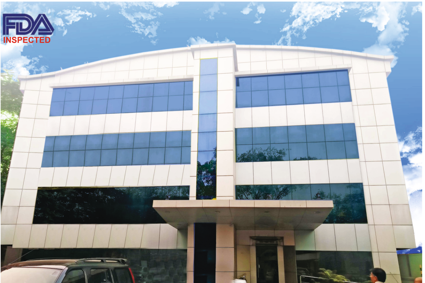
Maneesh Pharmaceuticals Ltd. - Mumbai, India Soft Gel Manufacturing Facility
